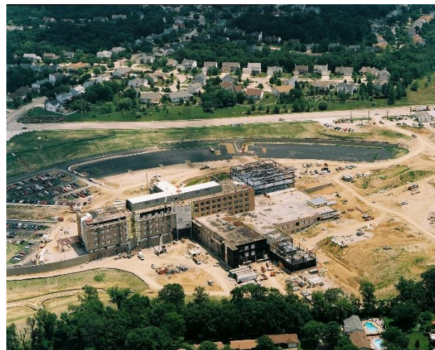
Figure 2: Aerial view showing proximity to residential areas
